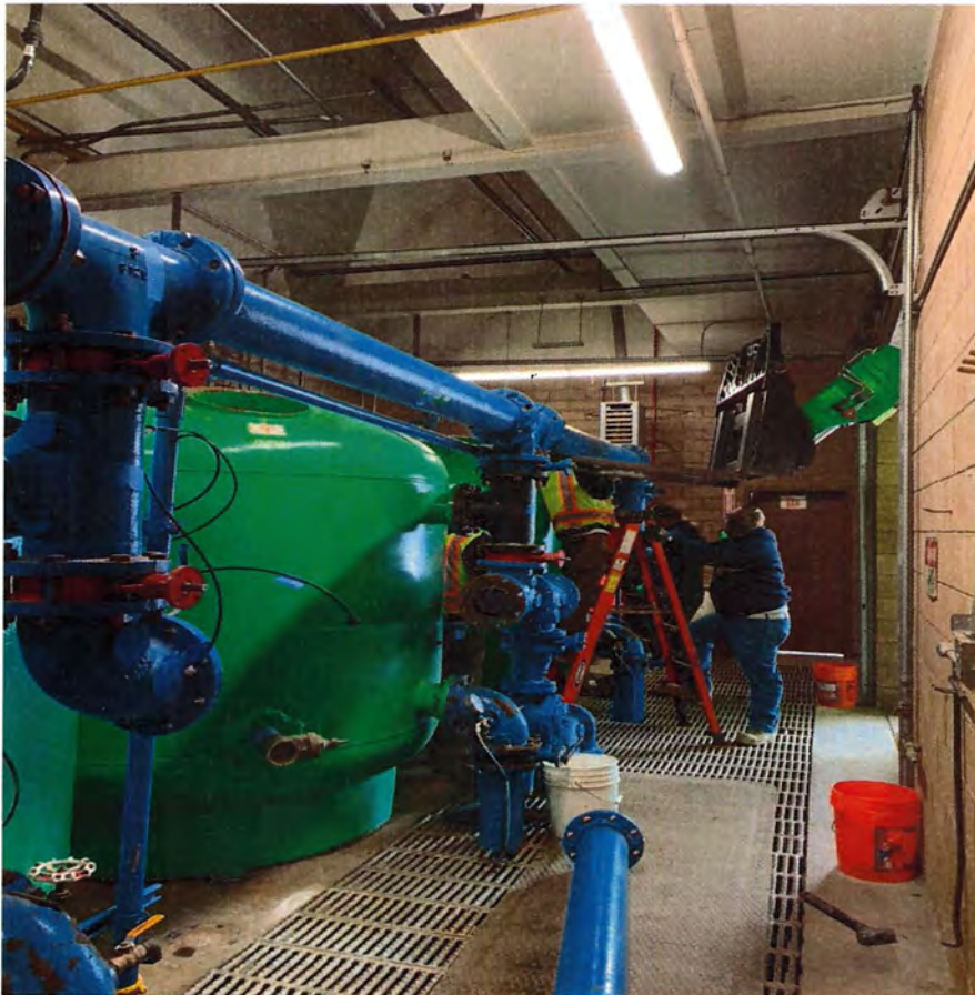
New Vessels in -Place with Manifold Piping Being Installed
